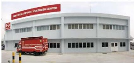
Hino Total Support Customer Center, a test drive and training facility for customers in Malaysia
